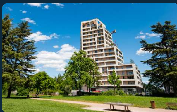
Plein Ciel • Strasbourg (67) Denu & Paradon Architecture
